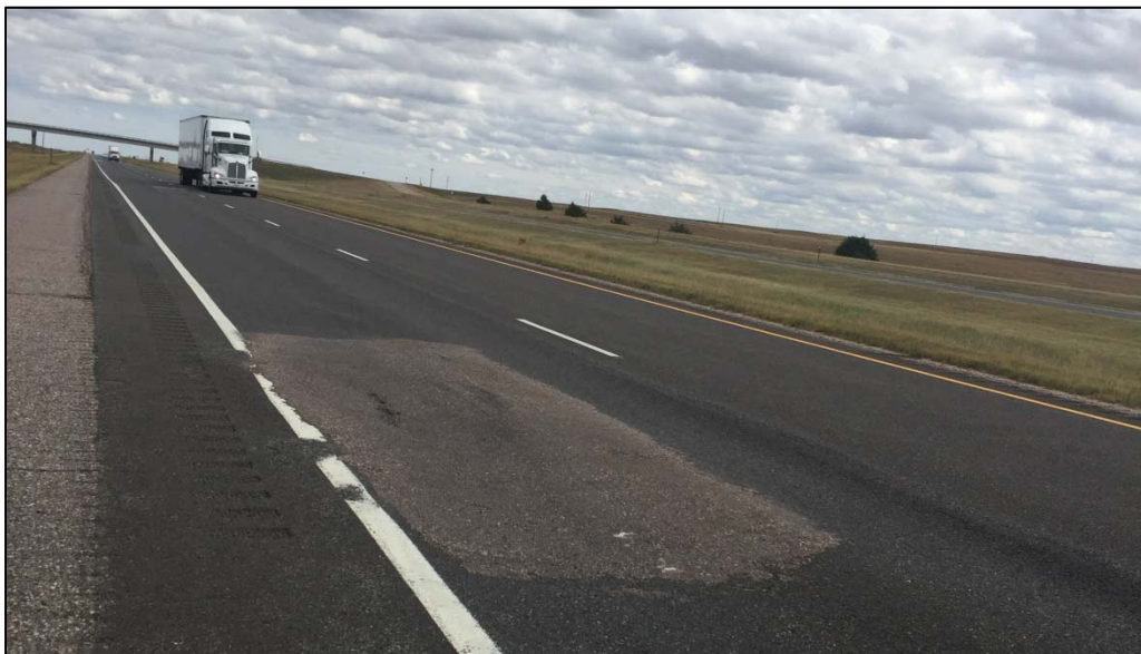
I-70 westbound lanes, looking east near Arriba interchange
